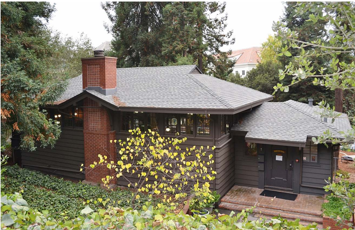
Girton Hall, UC Berkeley, built for Senior Women's activities in 1911, is listed on the California and National Register of Historic Places. This Morgan designed structure was relocated from its original site in 1946 and later adapted to its use as a day care facility.
